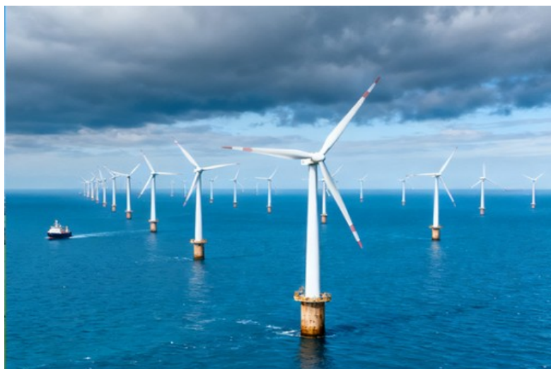
Figure I.5: Borssele Offshore Wind Farm [9].
